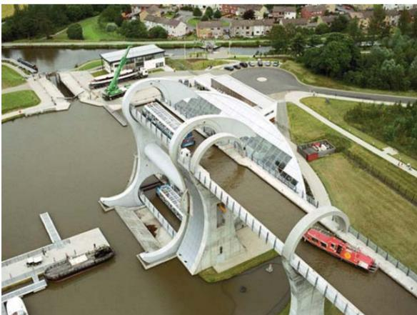
a boat enters, the amount of water leaving the caisson weighs exactly the same as the boat. This fundamental principle keeps the wheel balanced despite its enormous mass. Each caisson, whether empty or full, in effect weighs exactly the same. Rotating the wheel through the needed 180°, requires surprisingly little power. Just 22.5 kilowatts of power are needed for the five minute rotation, or about the amount of power needed to bake a loaf of bread in an electric oven.
